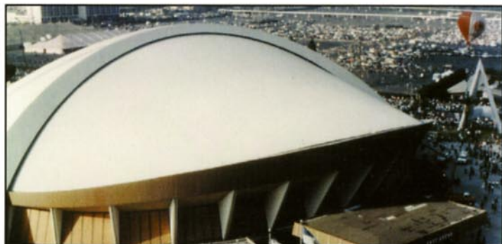
CONVENTION CENTER (after Re-Ply)
