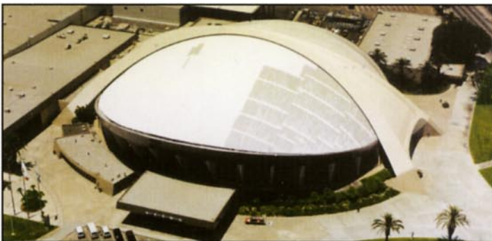
CONVENTION CENTER (metal roof)
