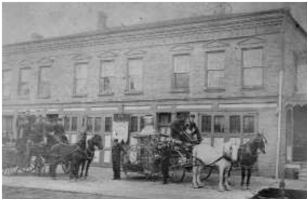
WAUKEGAN FIRE DEPARTMENT
