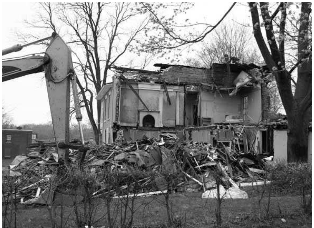
-Demolition of the Simmons-Cooke house, April 20, 2005 (Photo by Margaret Martin)
