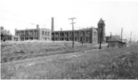
Southeast side of the Fansteel Plant. North Chicago, c. 1923.
