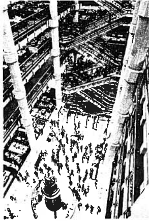
Lloyd's of London, view of concrete structure in atrium.
