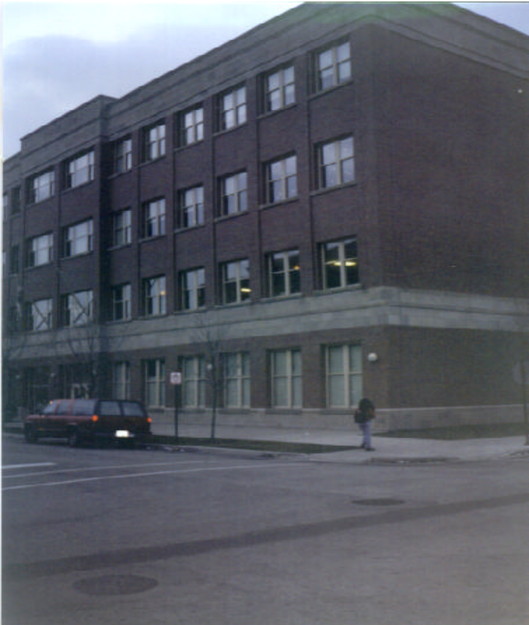
Figure 5. Gale School Annex near Northpoint, completed during the SECURE project.
