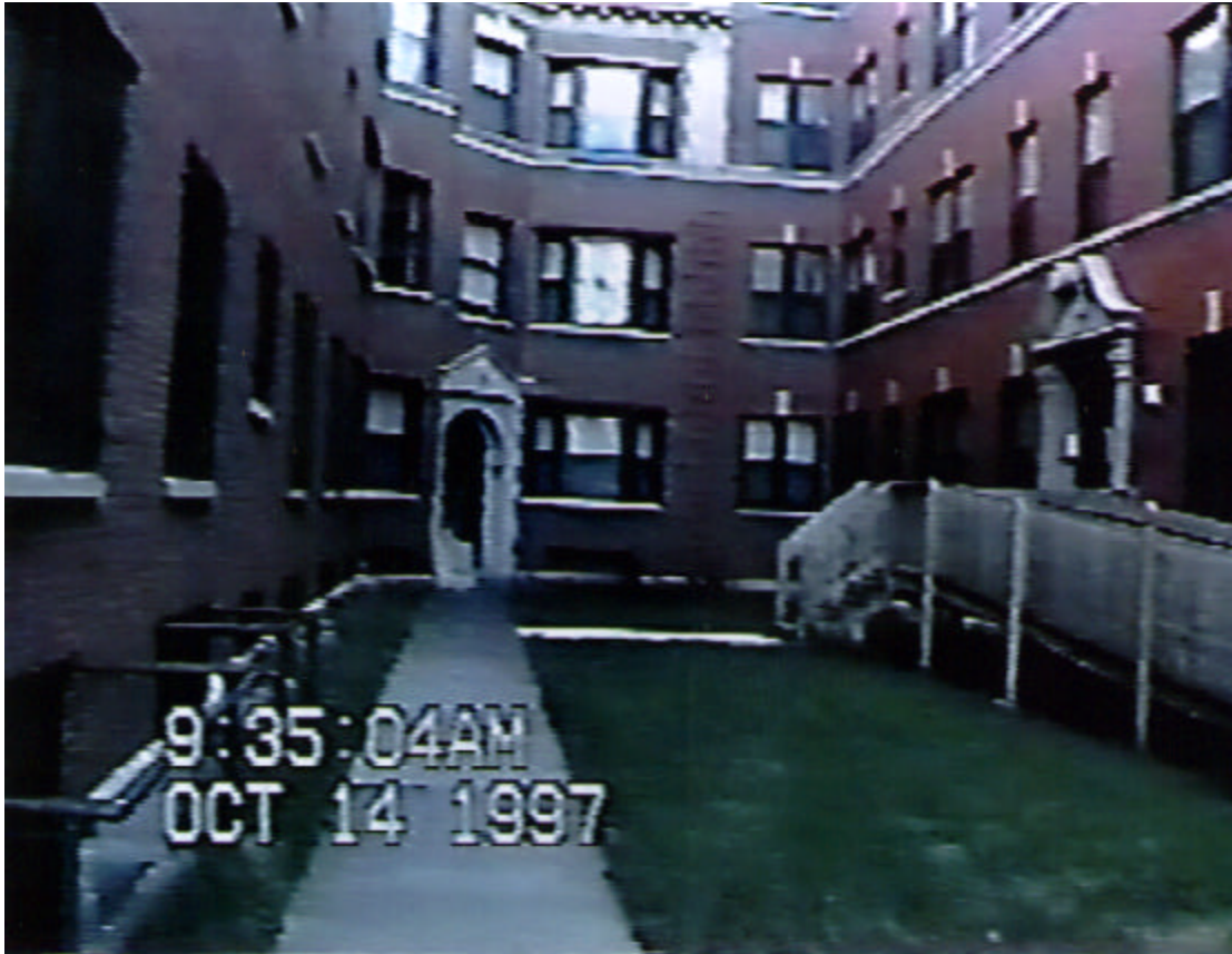
Figure 27. Park Apartments courtyard building.
