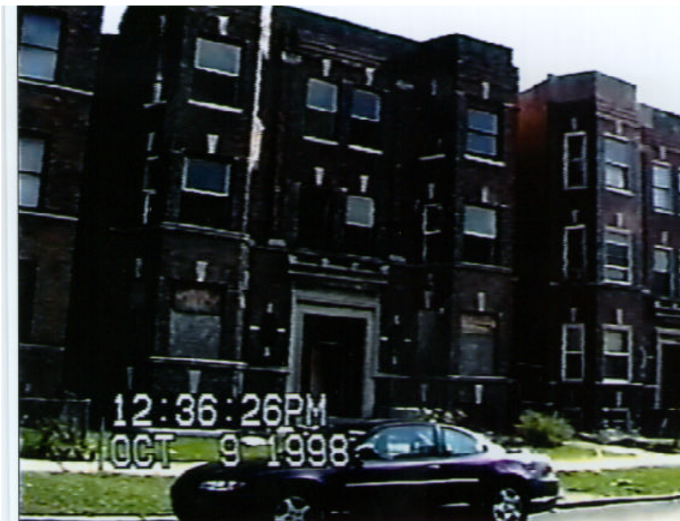
Figure 24. Abandoned building across the street from the Park Apartments building above. A young girl was recently found dead in this building.
