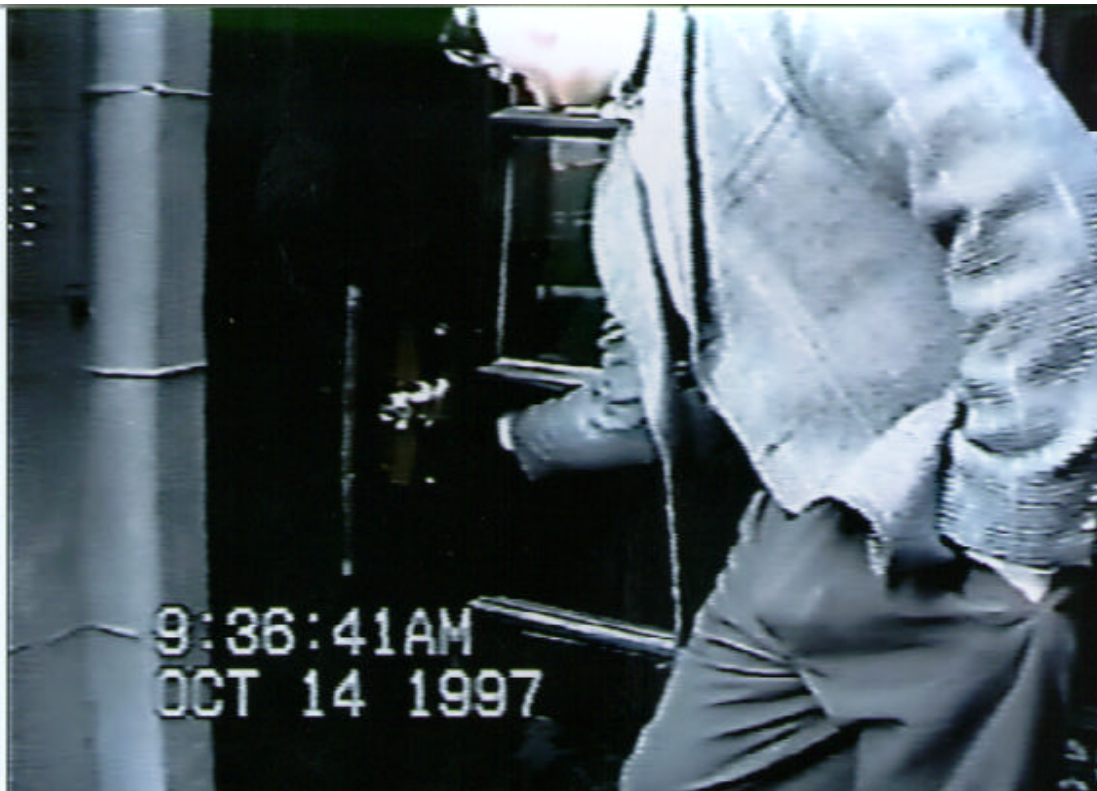
Figure 20. This door had a pane of glass broken, defeating the lock entirely.
