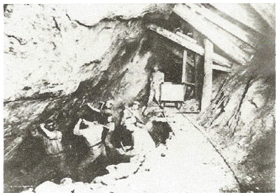
Wooden beams were used to support the shaft mine tunnels.
