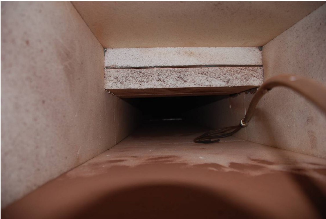
Figure 7 Duct cleaning using whip & compressed air
