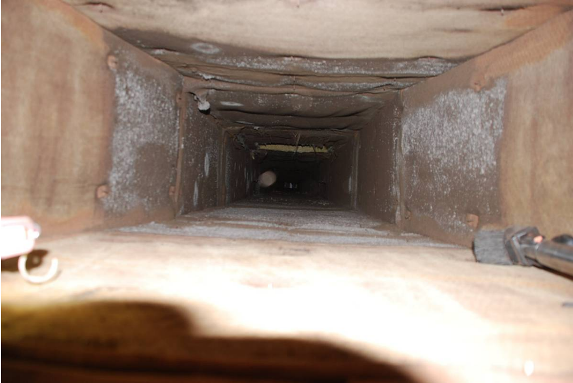
Figure 6 HEPA vacuuming of surfaces inside ducts
