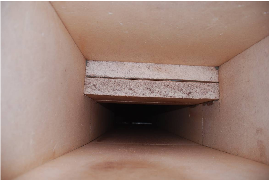
Figure 9 Duct cleaning using whip & compressed air
