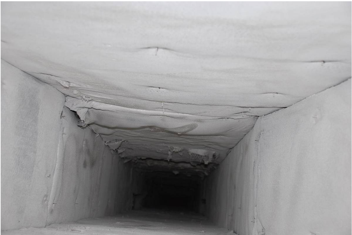
Figure 11 Encapsulation of ducting
