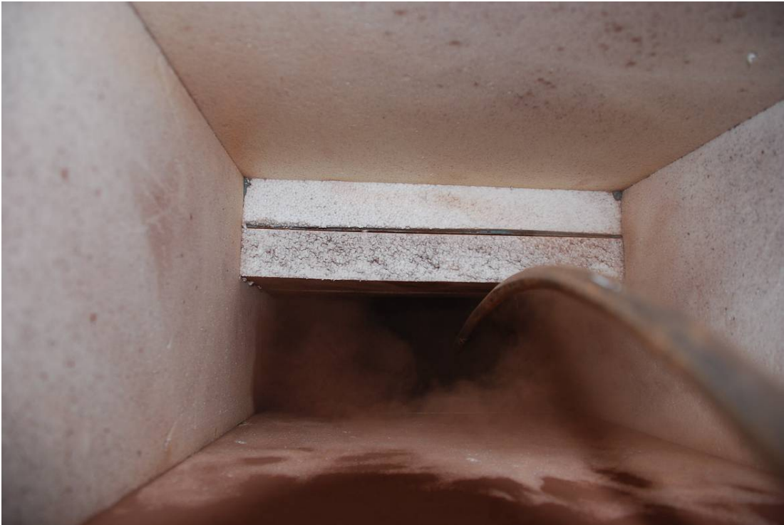
Figure 8 Duct cleaning using whip & compressed air
