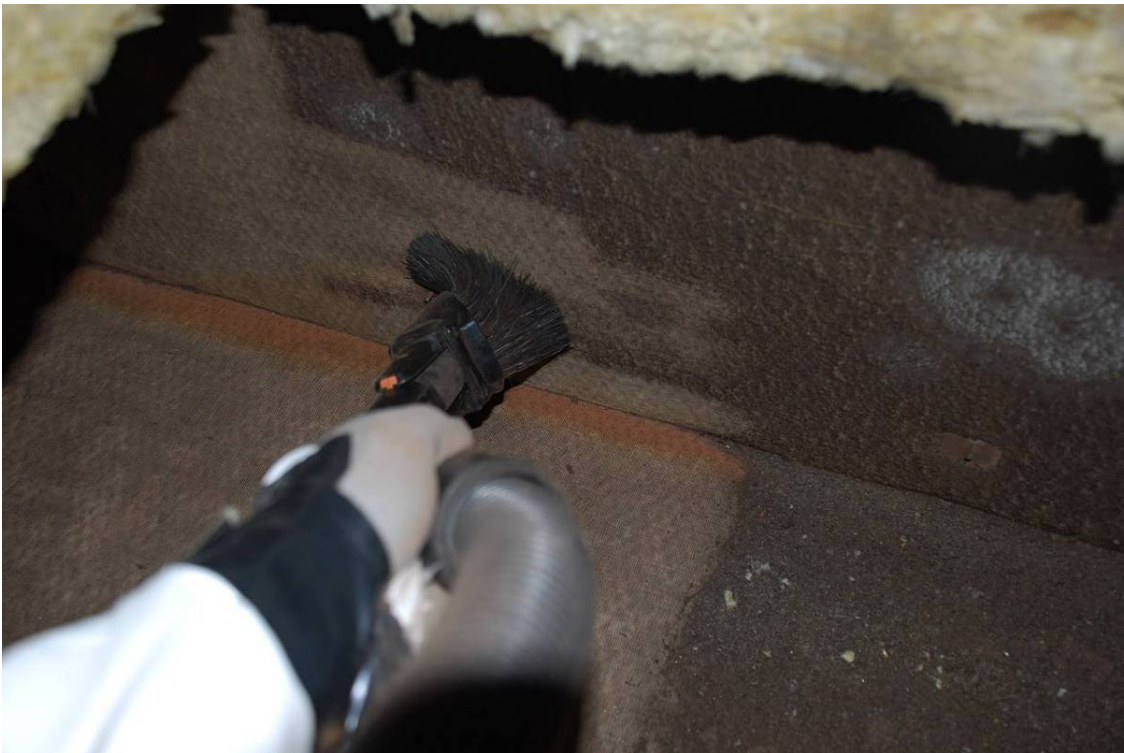
Figure 5 Contact cleaning inside ducts
