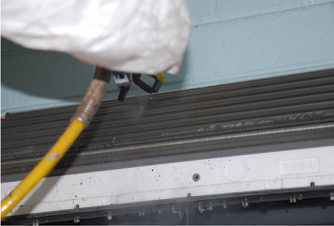
Figure 6 Remediation of cooling coils on split system HVAC
