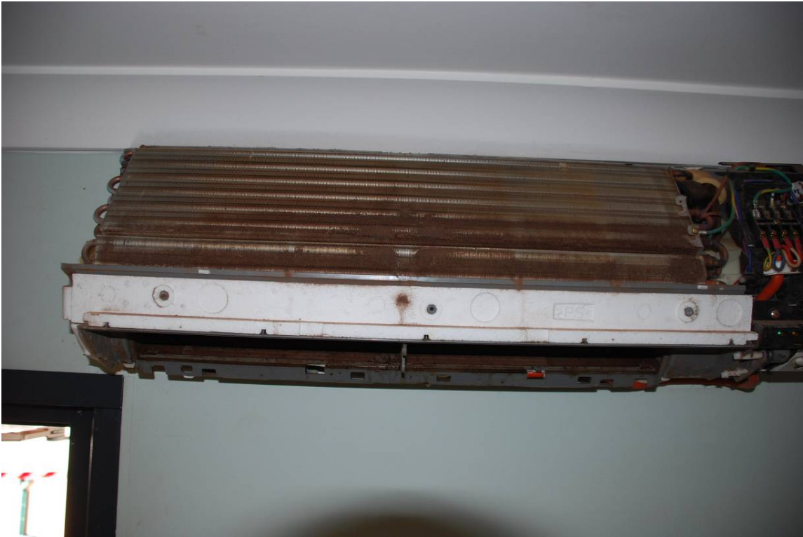
Figure 4 Cooling coils prior to hygiene & mould cleaning
