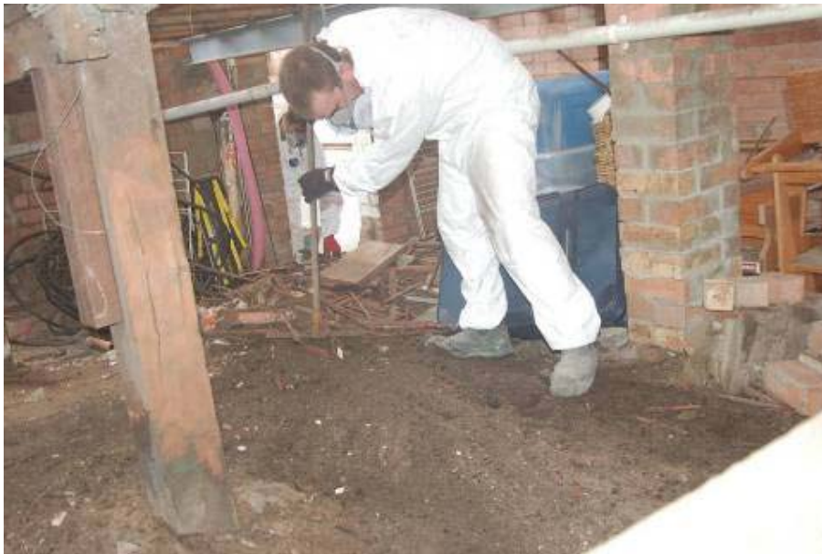
Figure 9 Remediation sub-floor soil
