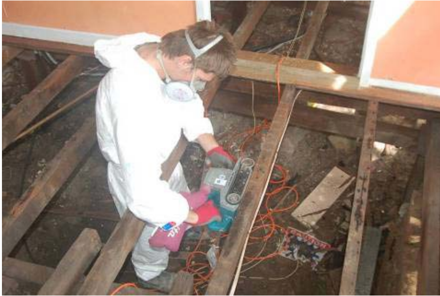
Figure 8 Sanding back of sub-floor timber
