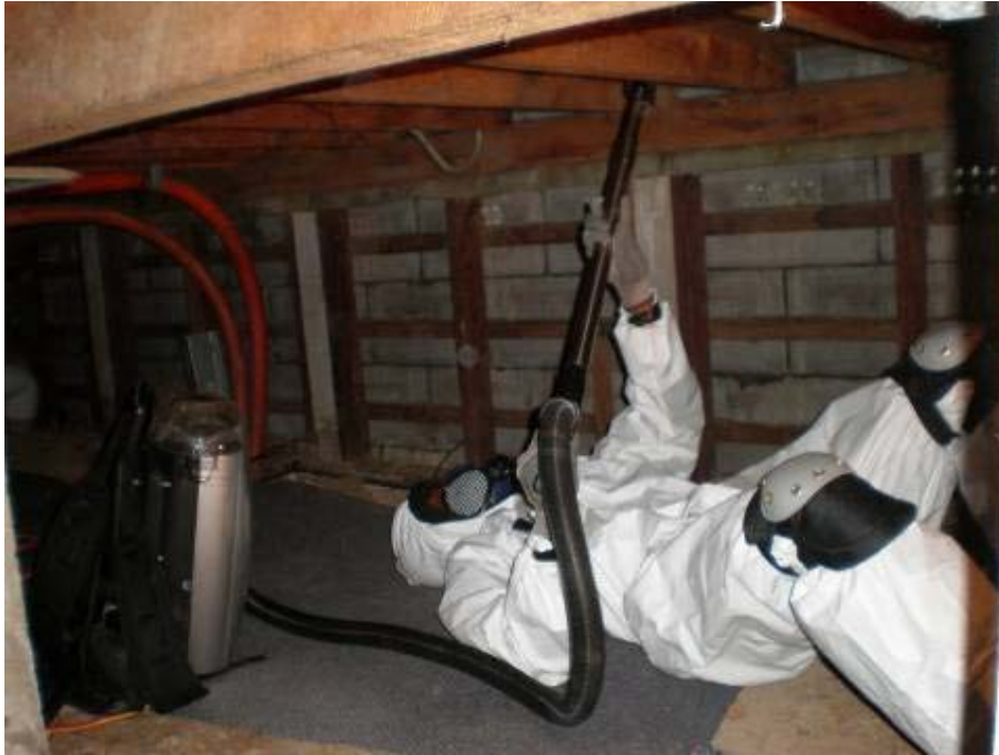
Figure 6 HEPA vacuuming
