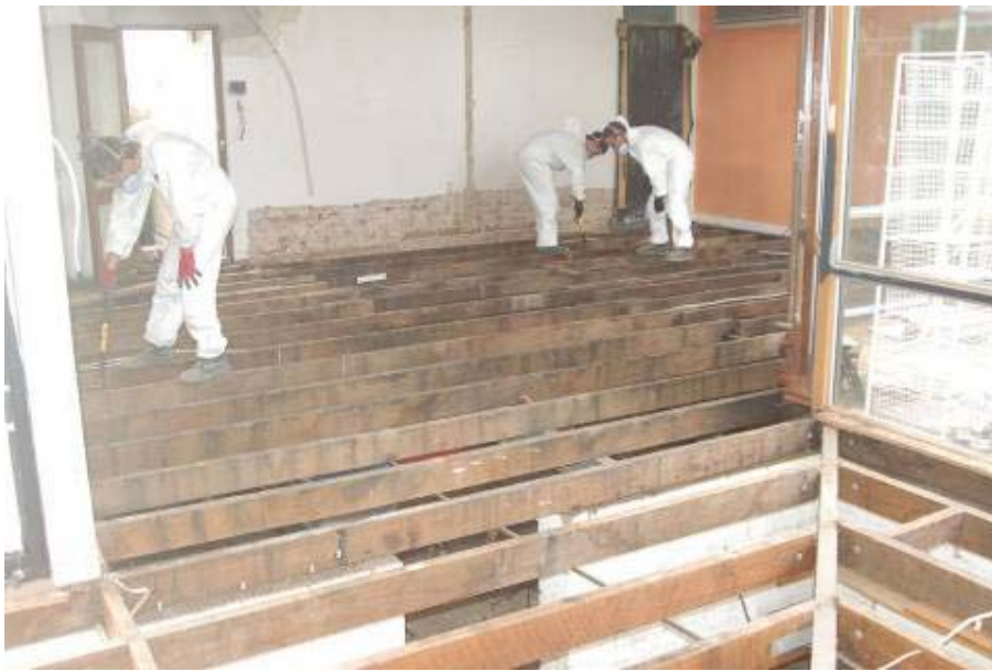
Figure 7 Removal of mould contaminated timber floor boards
