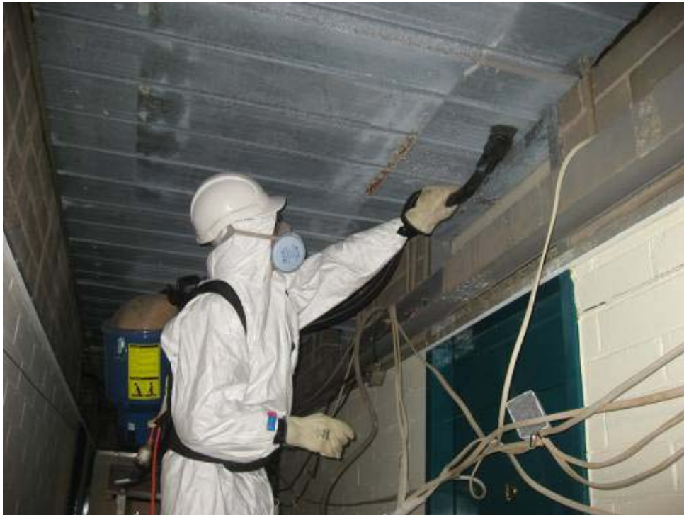
Figure 9 HEPA vacuuming
