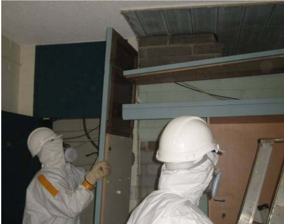
Figure 8 Removal of mould contaminated timber works
