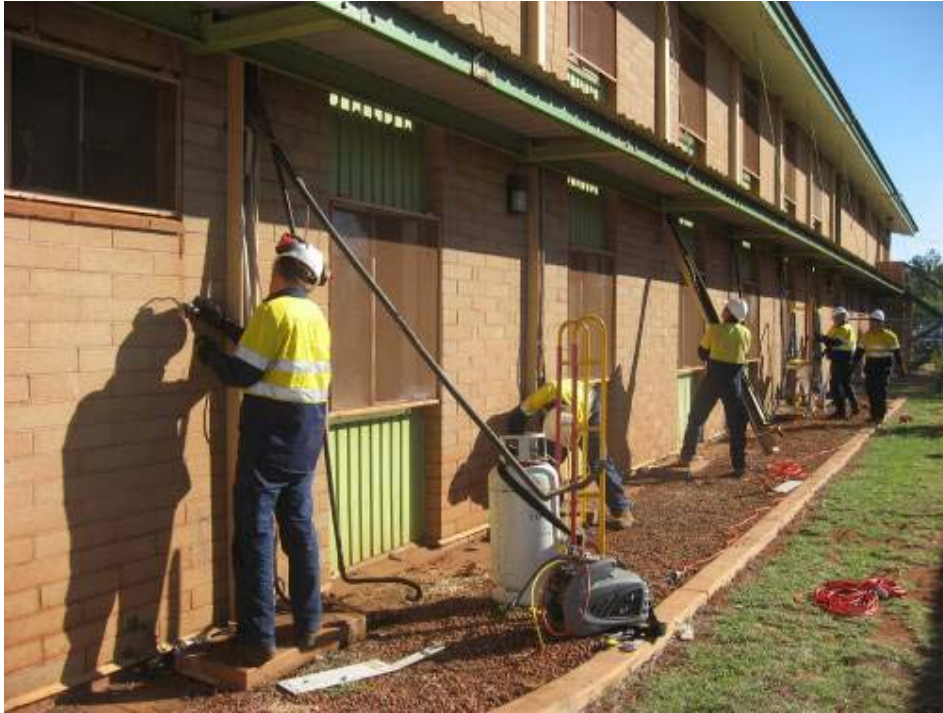
Figure 10 Re-installation of HVAC system
