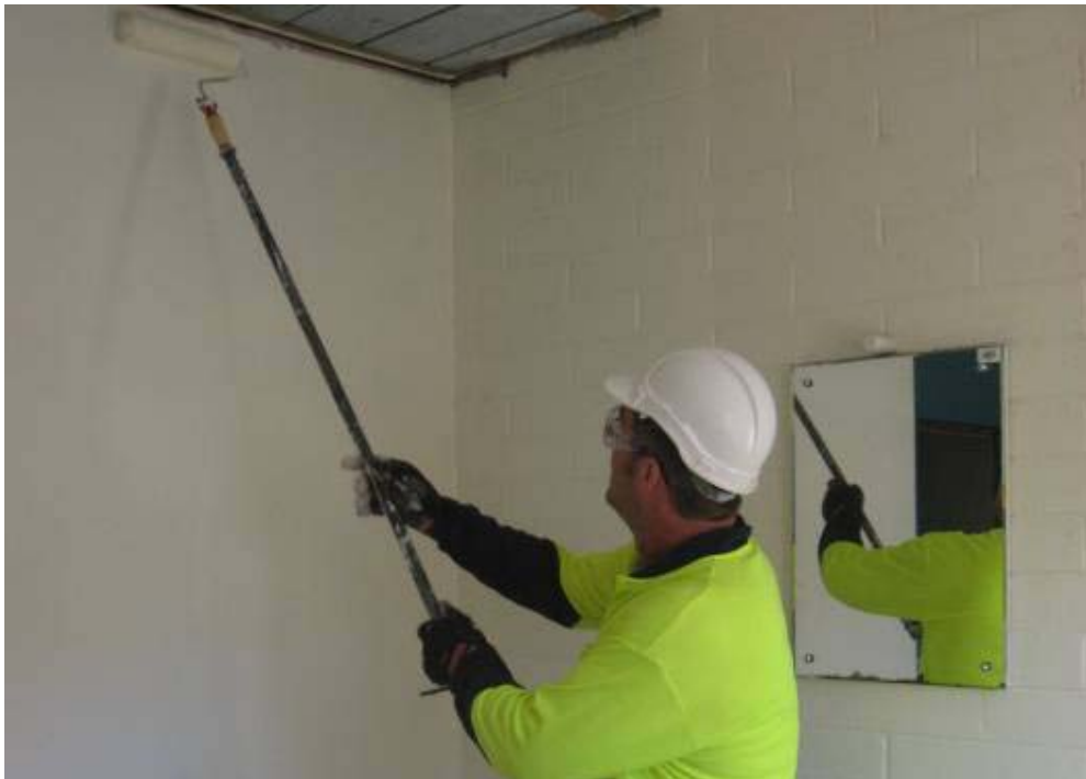
Figure 13 Painting of surfaces – walls and ceilings
