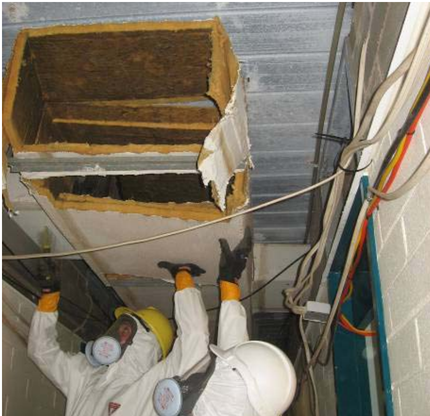
Figure 7 Removal of mould contaminated ducting
