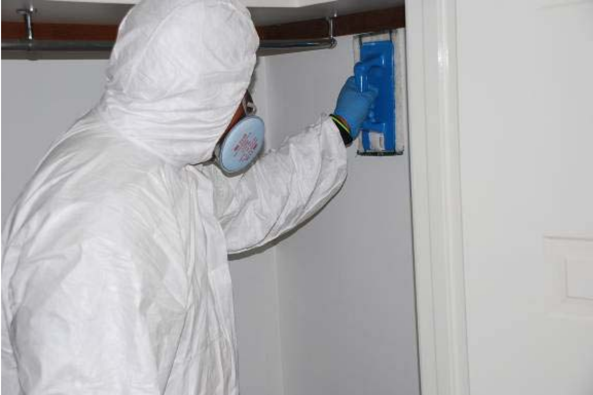
Figure 6 Damp wiping with micro-fibre cloth & mould cleaning solution
