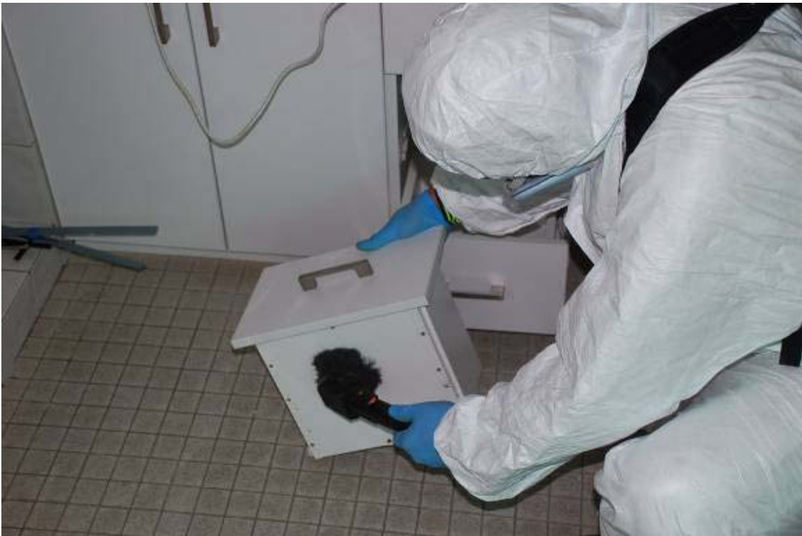
Figure 5 HEPA vacuuming of surfaces
