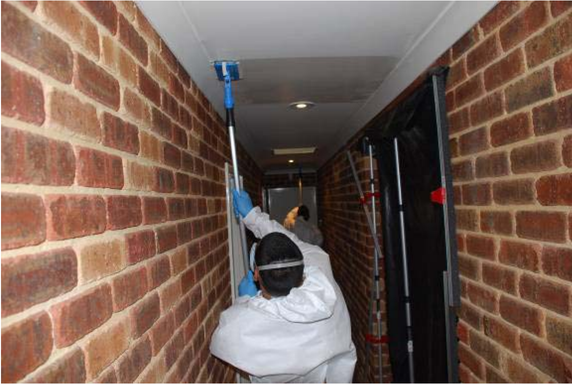
Figure 4 Remediation of ceilings with containment
