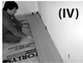
**PLEASE NOTE** that the stagger between the head joints should be 8" (20 cm) minimum, and preferably 12" (30cm). Cut the last planks of each row leaving a 3/8" (8-10mm) gap to the wall.
