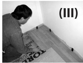
Do not attempt to knock the Uniclic® joint into place with one hit. Continue this method for each plank, covering the entire width of the room.
