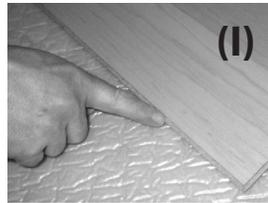
The cut piece from the first row becomes the starting piece for the second row. Install the cut edge facing the wall, with the expansion wedge in place. Now angle this piece and click it into the first plank of the first row. The cut pieces should be a minimum of 8" - 20cm in length (III).
