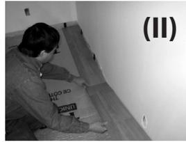
Continue the second row with a full piece, placing the tongue of the long side into the groove of first row piece (IV). Move the end joints together until they are approximately 1/4" - 6mm apart. Click the plank lengthwise into place. For the short edge, use a number of smaller taps with the Uniclic® tapping block, until the planks click into place completely.
