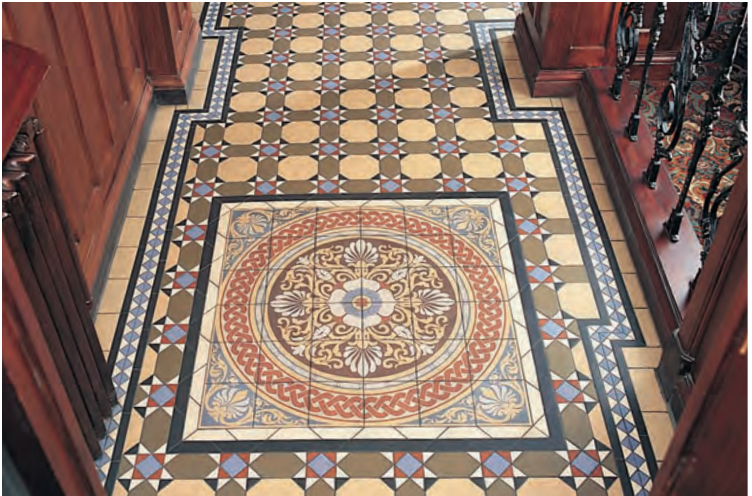
Above: Palmerston (Blue) used as centrepiece, framed by trapeziums, within Inverlochy pattern and bespoke border
