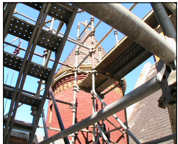
Church renovation begins.
