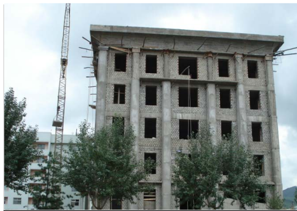
Construction on the Rajin branch of Golden Triangle Bank
