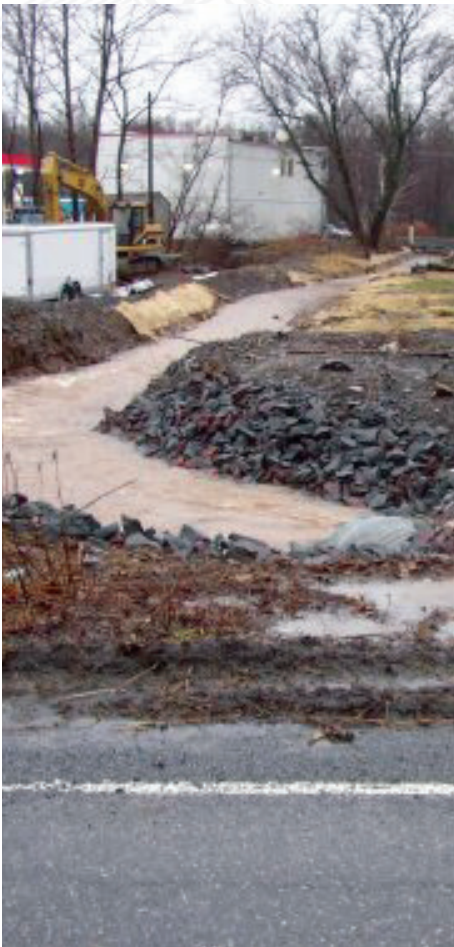
Without proper erosion control stormwater runoff from construction sites depletes topsoil and pollutes streams.
