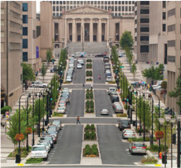
Deaderick Street, Nashville- Tennessee's first Green Street http://www.asla.org/uploadedFiles/CMS/Advocacy/Federal_Government_Affairs/Stormwater_Case_Studies/Stormwater_Case_242_Deaderick_Street_Renovation_(Green_Street),_Nashville,_TN(1).pdf
