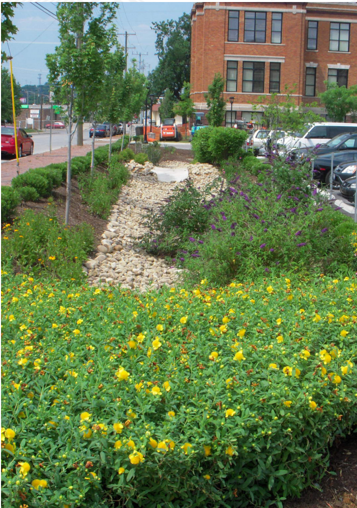
Case study of Bioswales at Metro's Richard H. Fulton Campus
