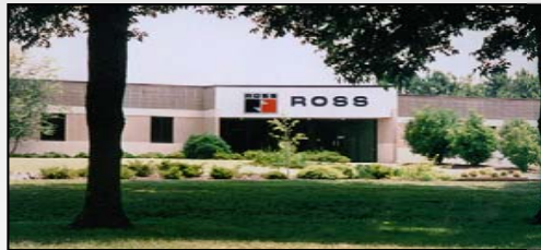
ROSS Controls - Lavonia, GA
