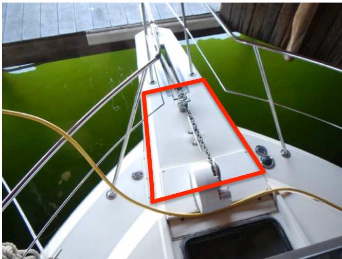
Pulpit structure is soft
