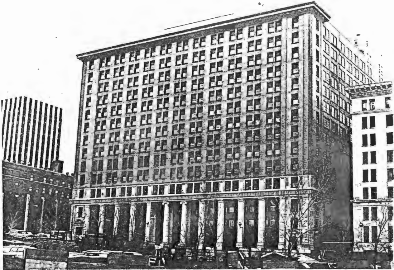
Lowertown Historic District, St. Paul, MN Railroad & Bank Bldg. (Burlington Northern Bldg.), 176 E. 5th St., South elevation
