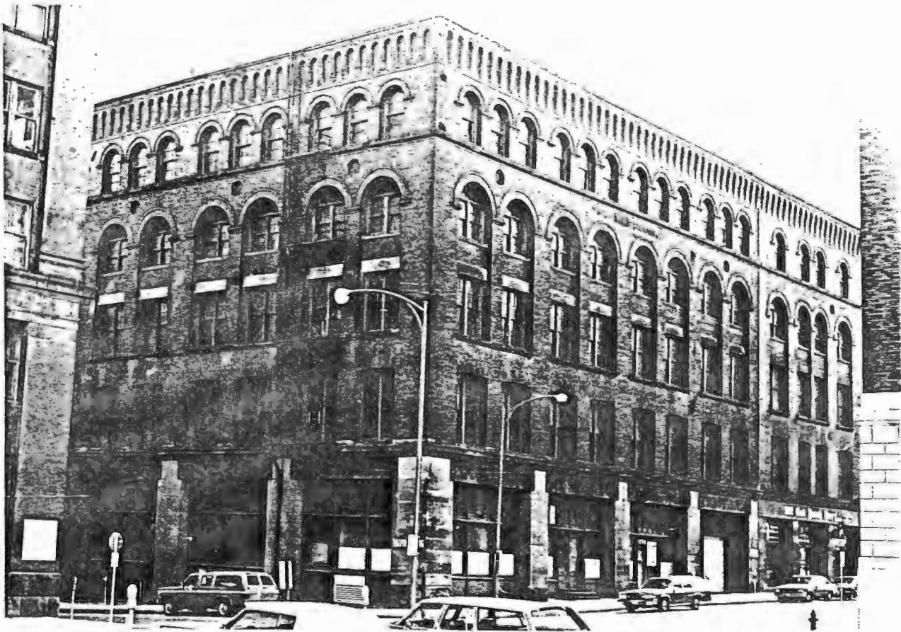
Lowertown Historic District, St. Paul, MN Hackett Block (Halper Bldg.) 262-270 E. 4th St. NE perspective 1982 No contact number (neg. at Ramsey Co. Historical Society)
