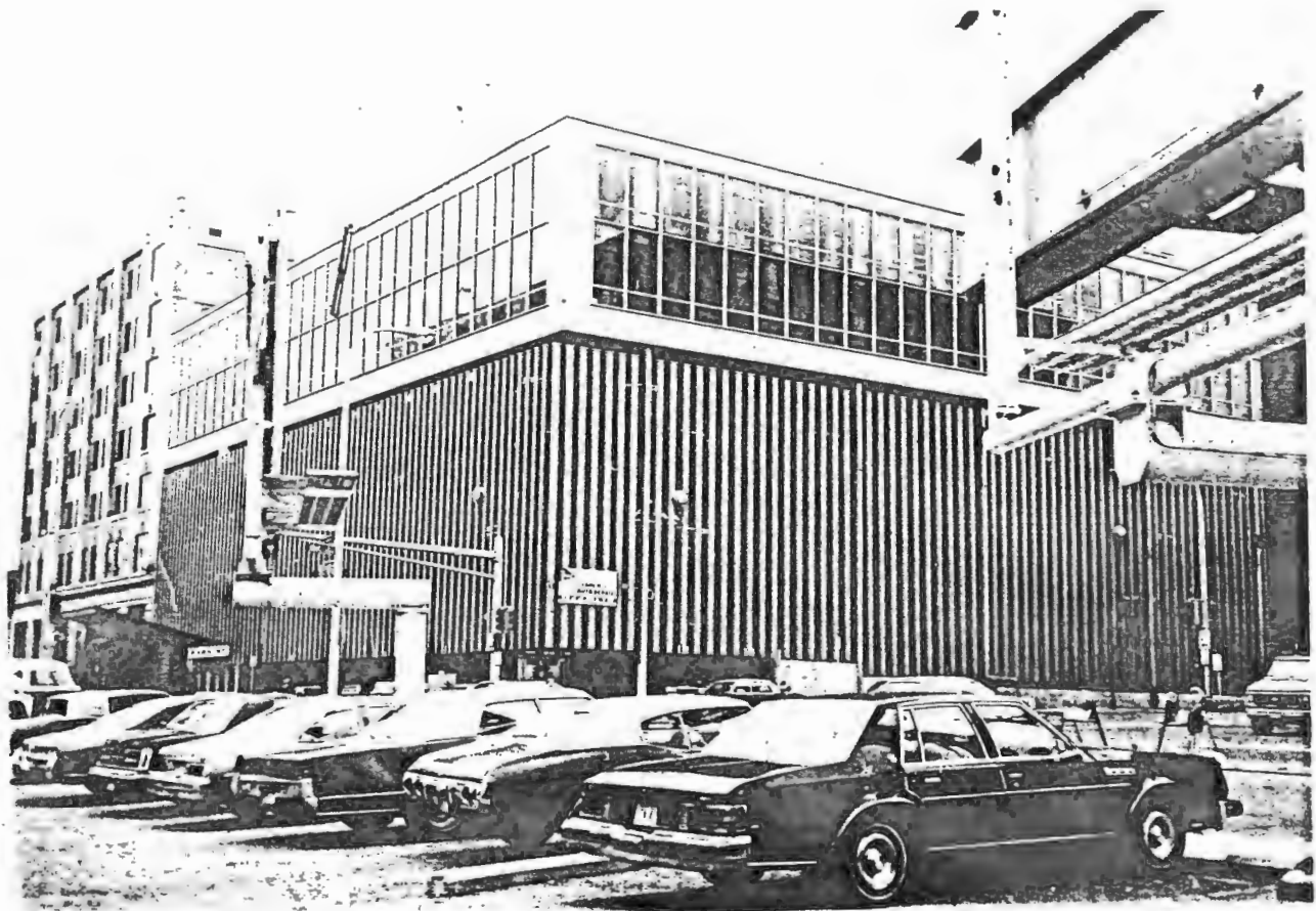
Lowertown Historic District, St. Paul, MN Control Data Business & Technology Center Garage, 245 E. 6th Street. Southeast perspective 1982 No contact number (neg. at Ramsey Co. Historical Society)
