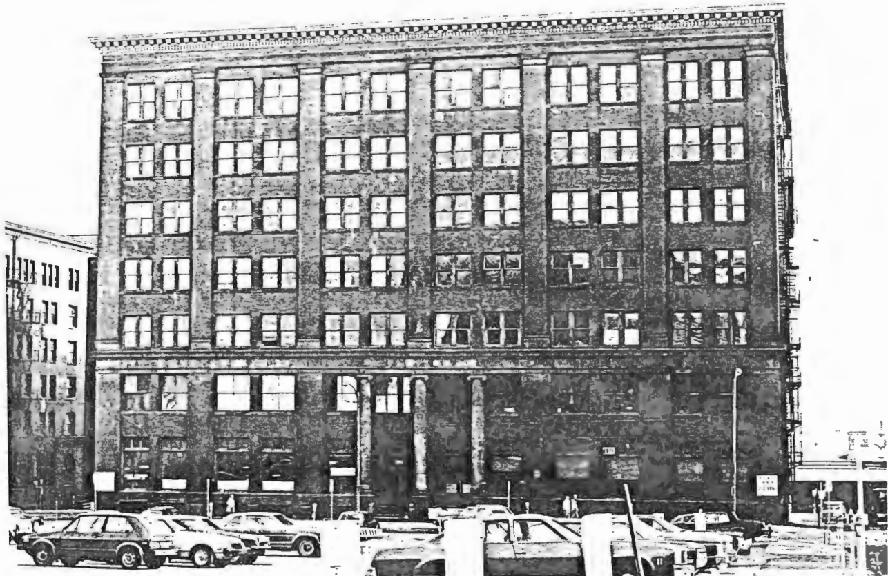
Lowertown Historic District, St. Paul, MN St. Paul Rubber Co. (E.W. Honza Printing Co.), 300 E. 4th Street, North elevation
