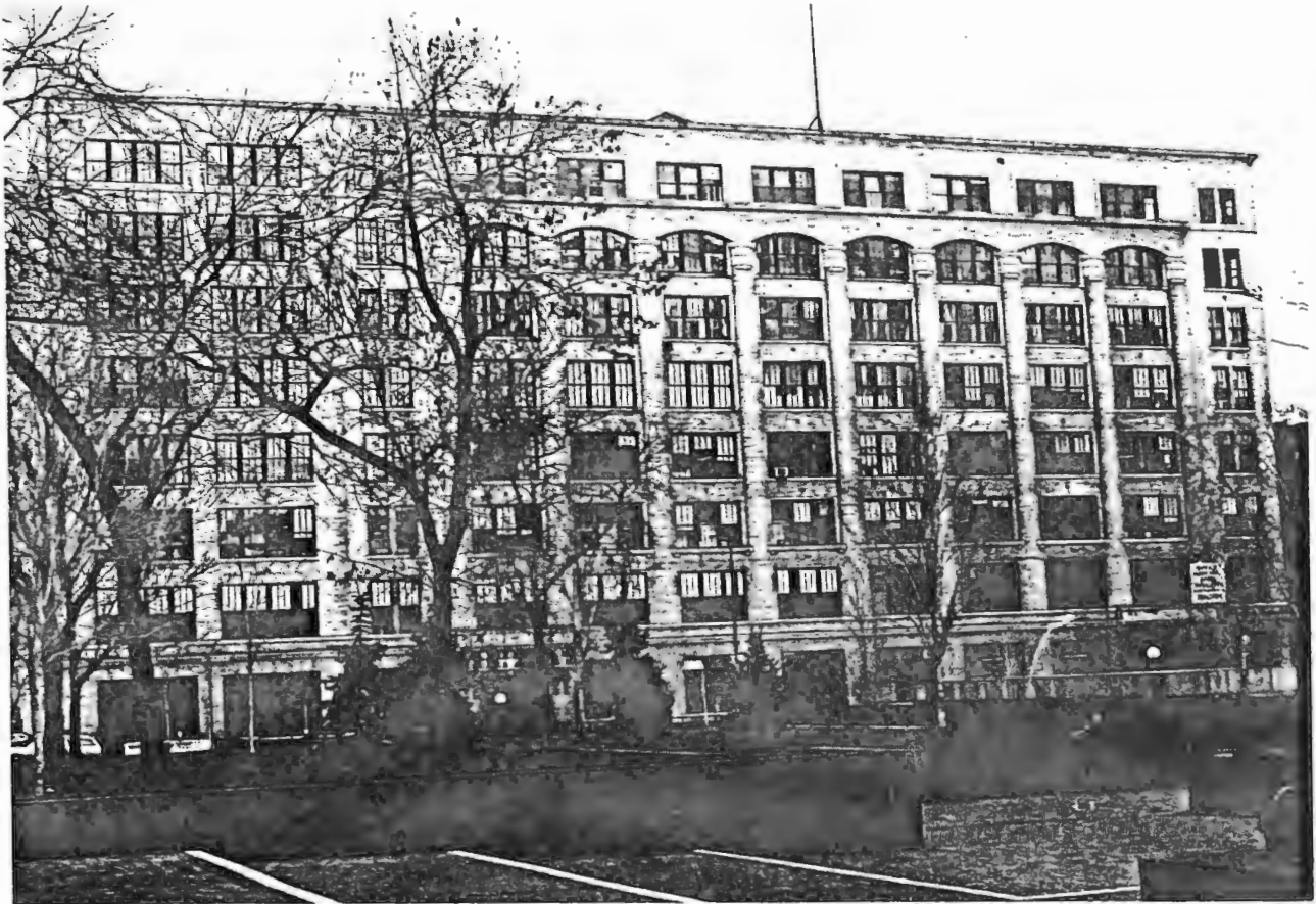
Lowertown Historic District, St. Paul, MN Finch, VanSlyck & McConville Dry Goods Co. (Finch Bldg.), 366 Wacouta St, West elevation 1982 No contact number (neg. at Ramsey Co. Historical Society)
