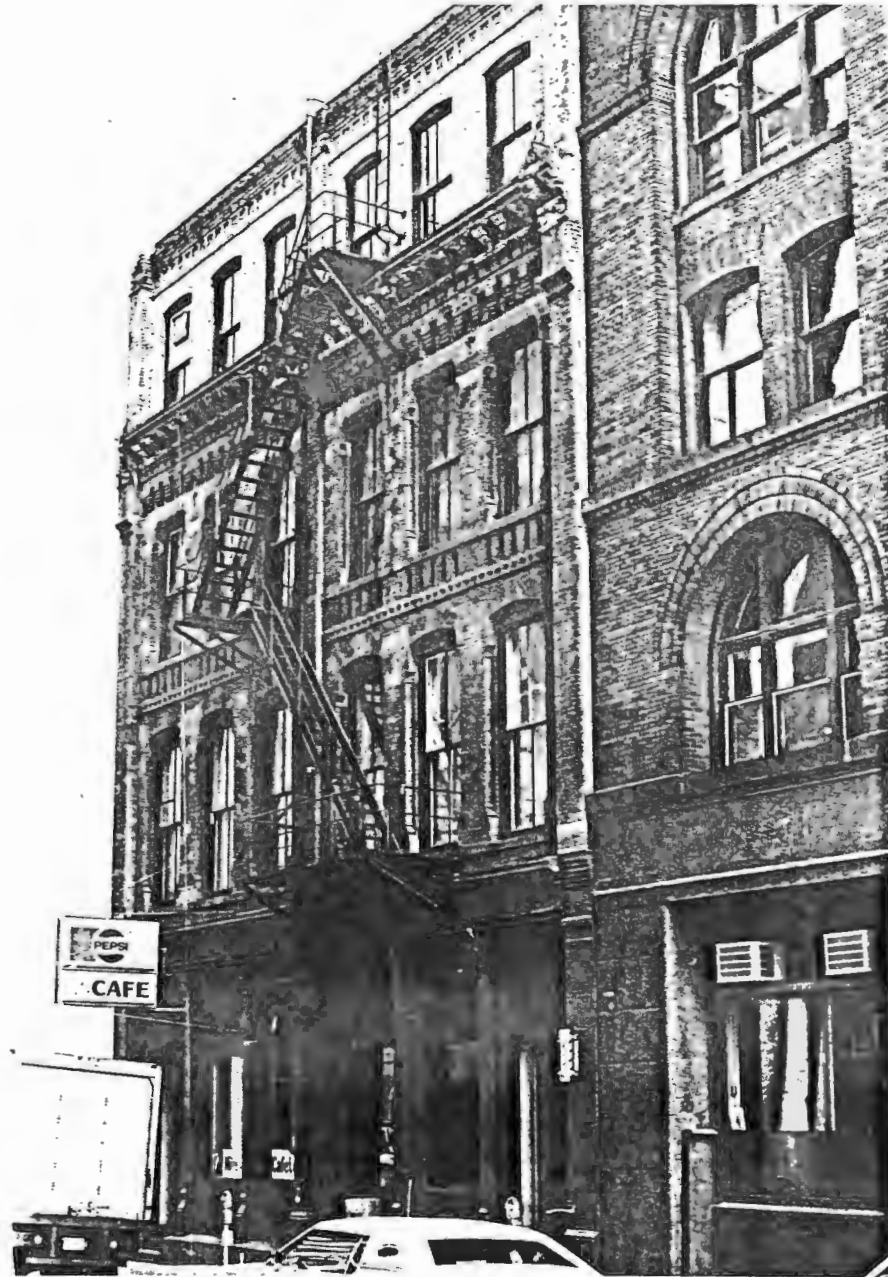
Lowertown Historic District, St. Paul, MN Mike & Vic's Cafe, 258-260 E. 5th Street, North elevation 1982 No contact number (neg. at Ramsey Co. Historical Society)
