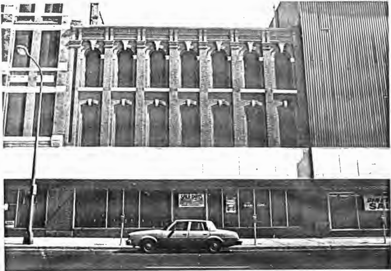
Lowertown Historic District, St. Paul, MN Walterstroff and Montz Bldg. (Butwinick's Furniture), 216-220 E. 7th St. North elevation 1982 No contact number (neg. at Ramsey Co. Historical Society)
