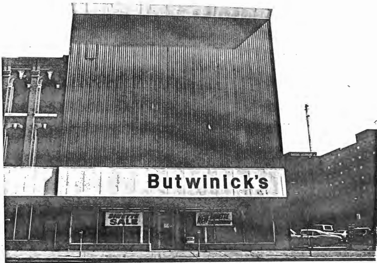
Lowertown Historic District, St. Paul, MN J.H. Weed Bldg. (Butwinick's Furniture), 208-212 E. 7th St., North elevation 1982 No contact number (neg. at Ramsey Co. Historical Society)
