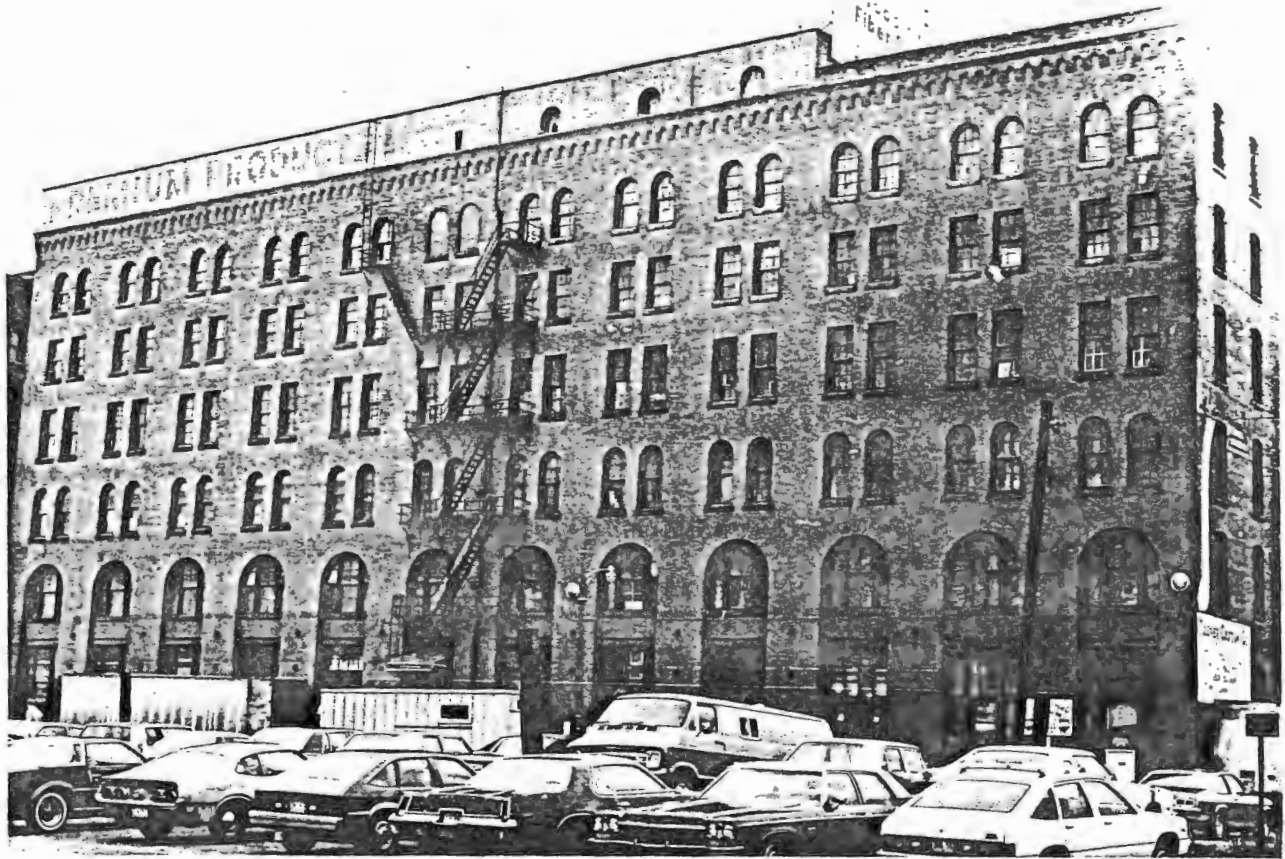
Lowertown Historic District, St. Paul, MN Griggs & Foster's Farwell, Ozmun & Kirk Bldg., (Tilsner Carton Co.), 300 Broadway Street. North elevation
