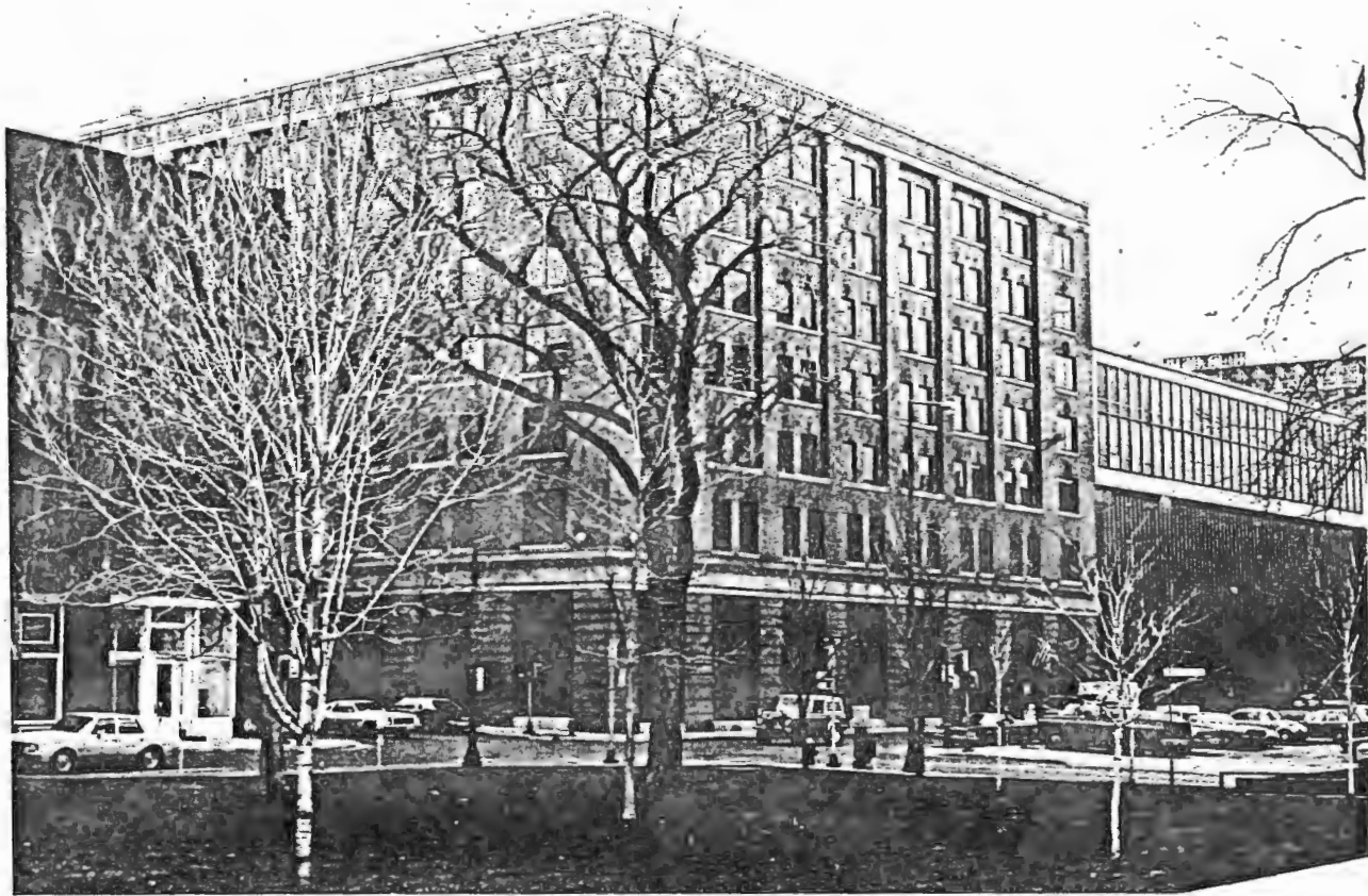
Lowertown Historic District, St. Paul, MN George Sommers & Co. Bldg. (Control Data Business & Technology Center), 245 E. 6th Street. Southwest perspective 1982 No contact number (neg. at Ramsey Co. Historical Society)
