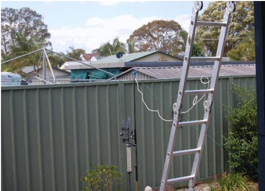
Initial set-up at ground level.
