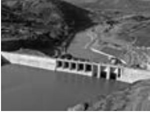
Devecikonağı HES SSB Baraj H = 40 m
