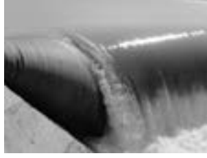
Azmac HES Lastik Savak L= 48 m, Q = 1000 m 3 /s
