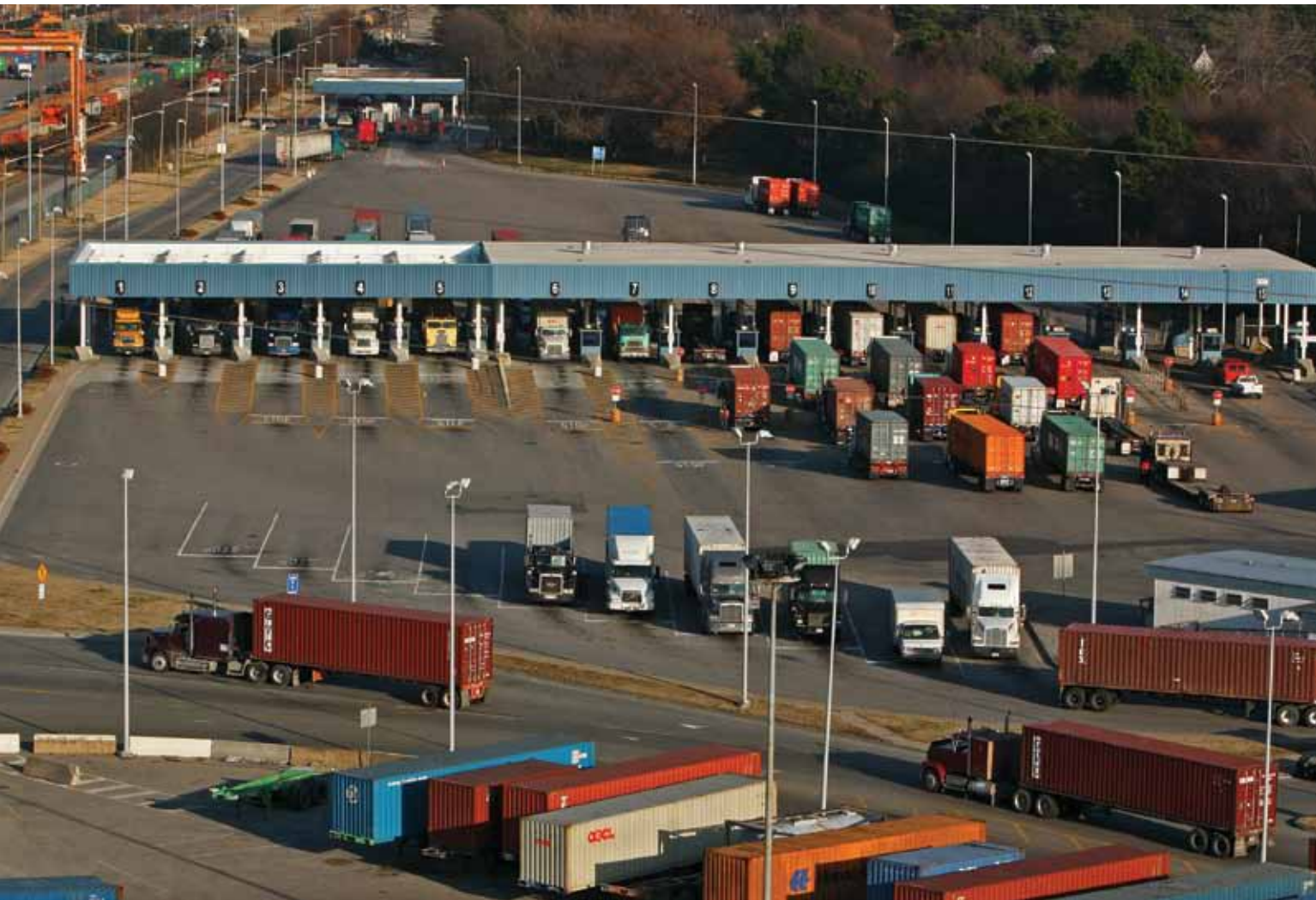
VIRGINIA PORT AUTHORITY
