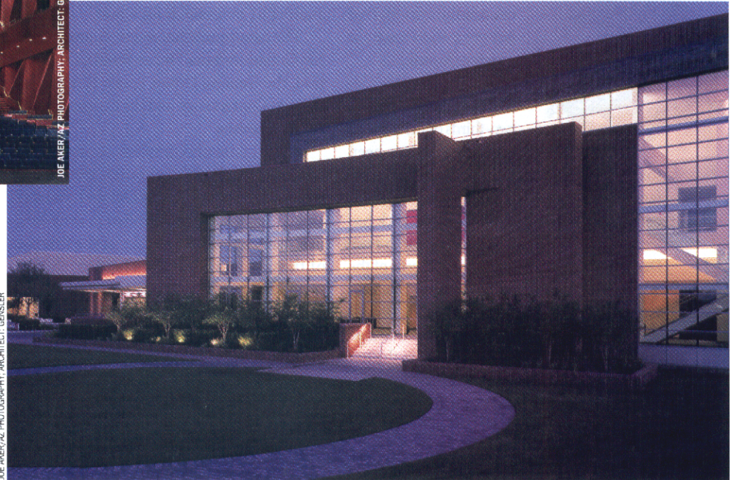
JOE AMER/AZ PHOTOGRAPHY; ARCHITECT: GENSLER
