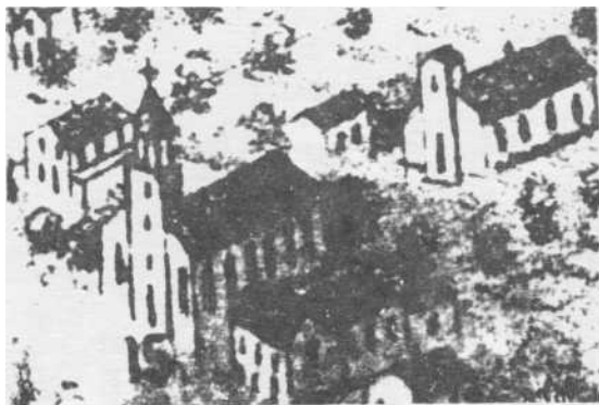
The St. Francis de Sales Church Complex in 1870 indicating the Church and Rectory Lamy built in 1842.
