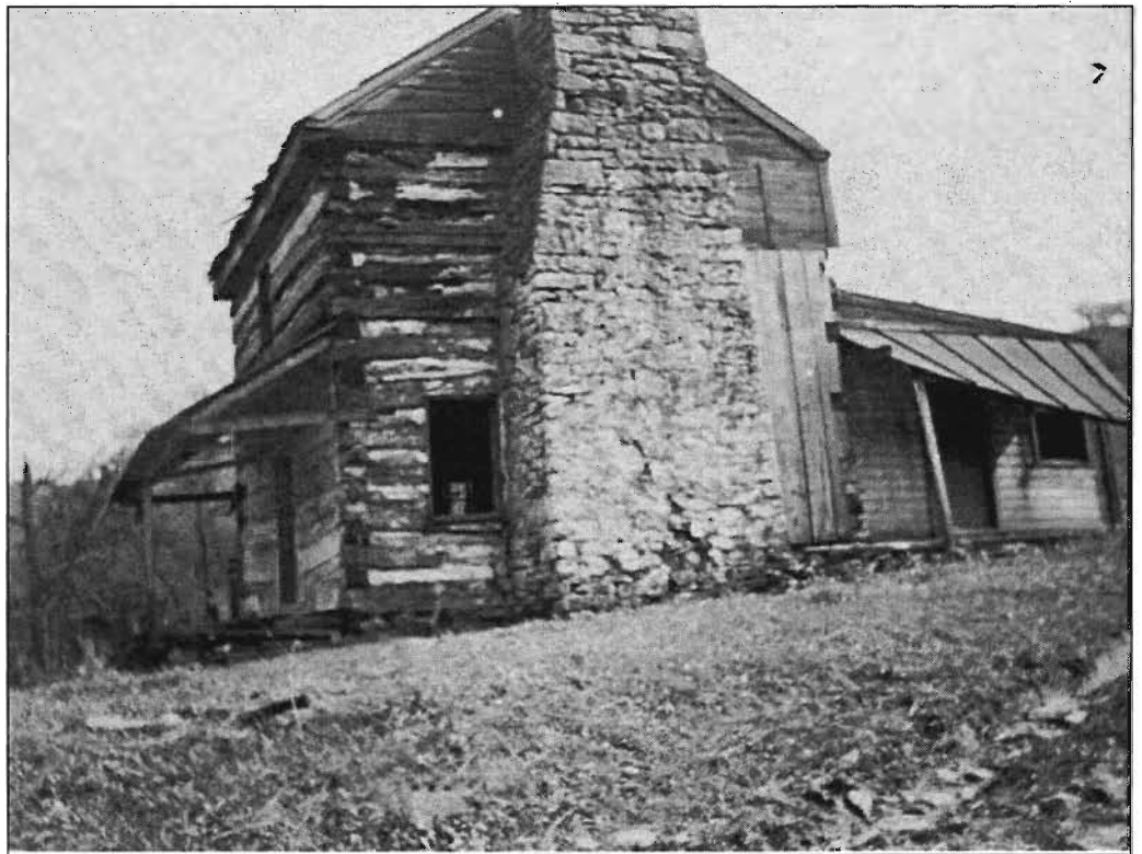
A cabin in Granville, Ohio's Welsh Hills.
