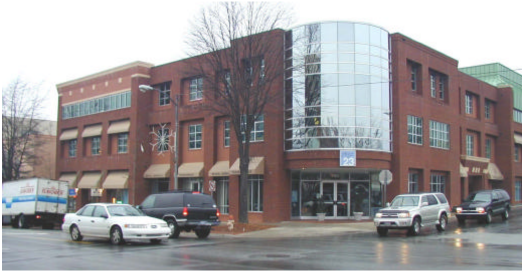
New construction on West Franklin Street.
