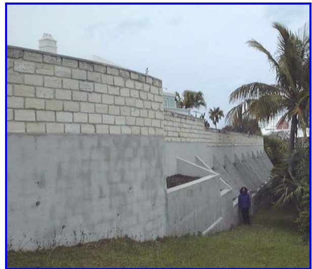
Plate 30. Two years after completion, the planters in the 15 ft. high boundary wall on this residential property remain bare. (Photo from Bermuda Biodiversity Project).
