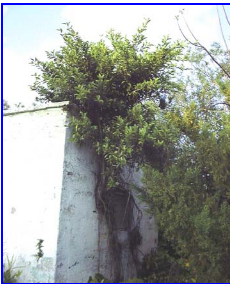
Plate 22. The invasive Indian Laurel tree growing out of the side of a building. (Photo courtesy of H. De Silva).
