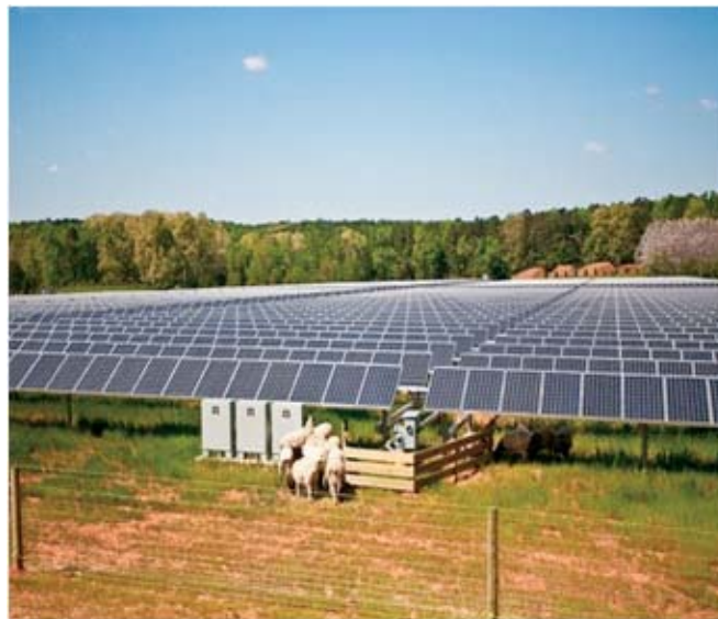
Figure 19. Solar panel array.
